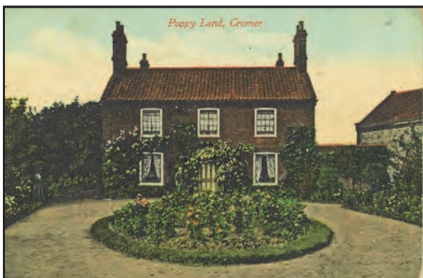
Fig 5 The Mill House
